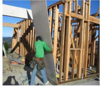
Blazeguard Panels being installed in Carmel, CA
