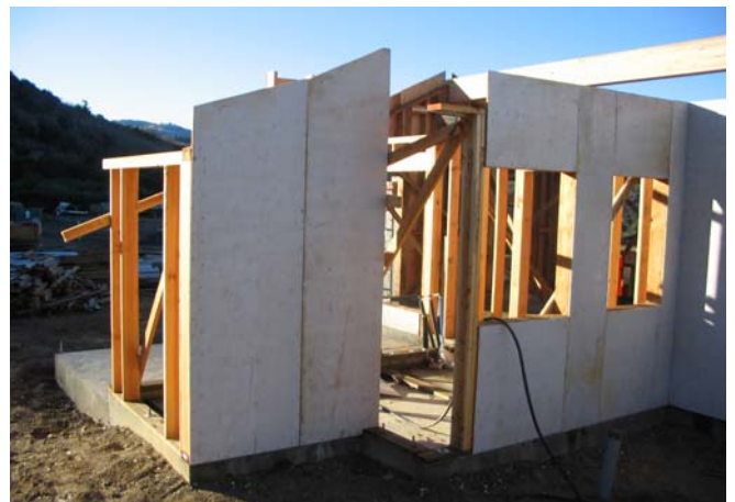
Blazeguard provides a fire barrier as well as structural sheathing in a single, environmentally friendly panel.
