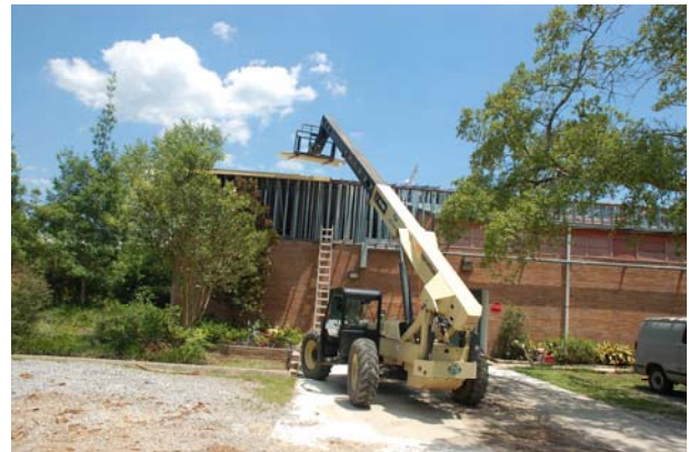
Blazeguard® Fire-Rated Sheathing is lifted to the rooftop of the school for new roof construction.
