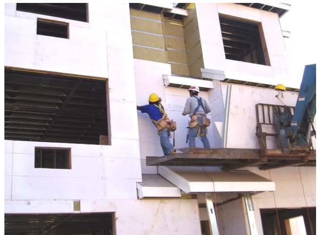
Workers apply Blazeguard (white face) sheathing using standard construction tools and practices.
