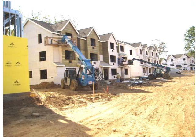
Blazeguard® Fire-Rated Sheathing will protect all exterior walls on these buildings at Markham Gardens in New York.
