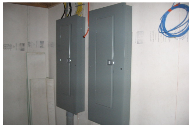
Blazeguard® serves as a fire-resistance-rated panel backer board for behind electrical panels.
