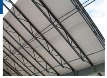
Blazeguard ® (white face) protects the inside face of these commercial SIP roof panels in Ohio
