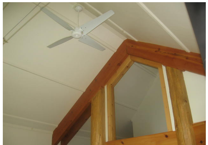
Interior SIP ceiling/roof surfaces can be painted and seams hidden with battens for a finished look.
