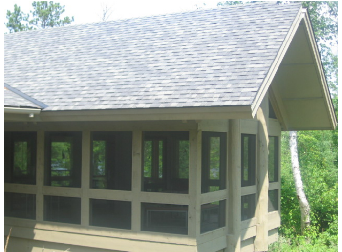
Blazeguard® coated SIPs allow this lake cabin to be “off-grid” and heated/cooled locally and naturally.
