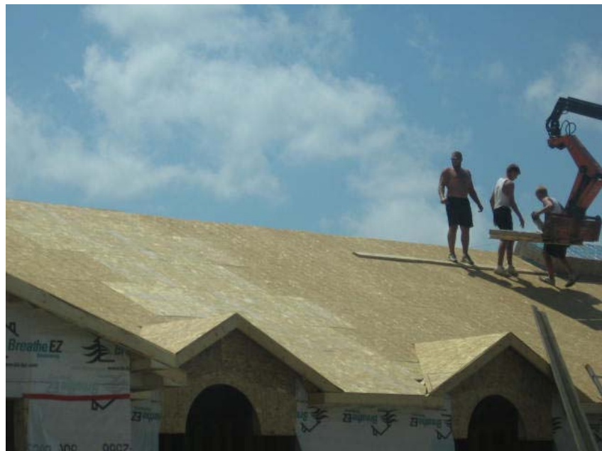
Figure 3: Blazeguard (lighter colored boards) as seen from the rooftop.
