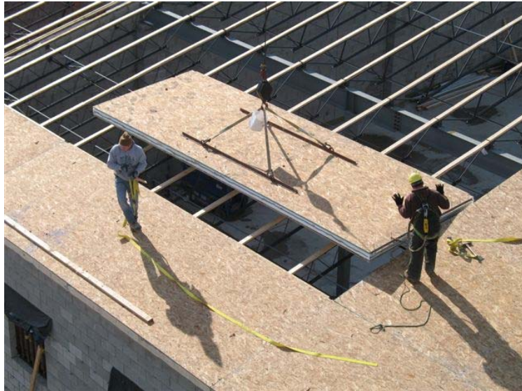
Figure 1: Workers place an 8' x 24' jumbo SIPs panel in Marysville, Ohio.
