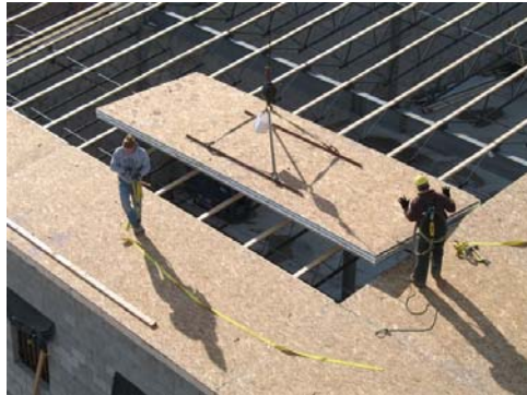
Workers place a Jumbo SIP panel.
