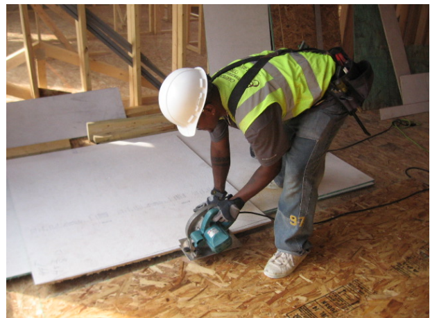
Blazeguard sheets can be cut and nailed into place using standard construction tools and techniques.
